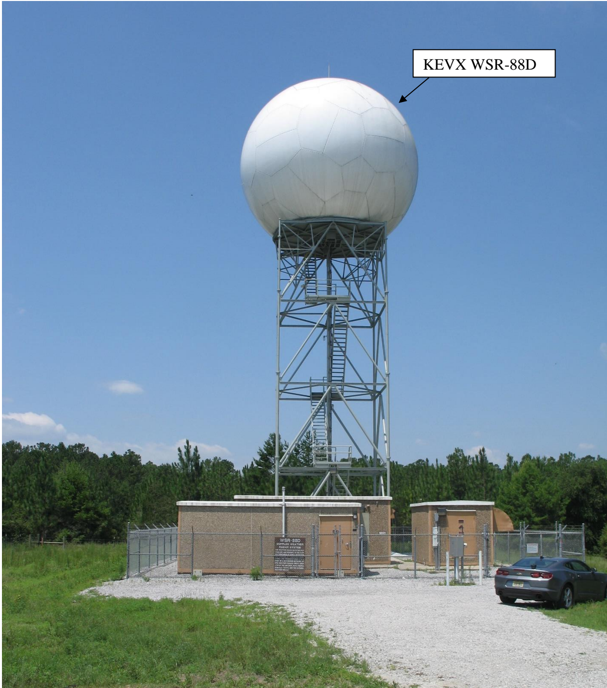
Figure 1: Photograph of KEVX WSR-88D serving Eglin AFB, FL, area
