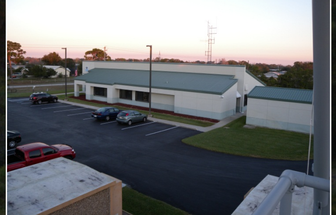
KMLB Tower View to Northwest
